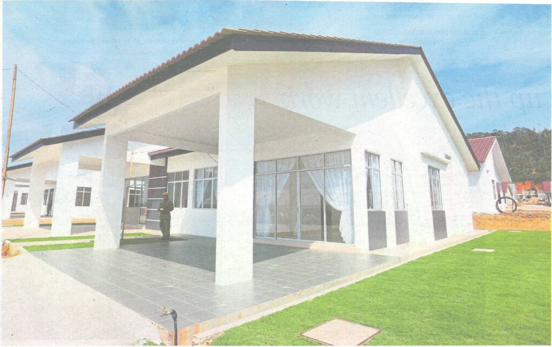
The 1Malaysia People's Housing Programme (PRIMA) is championing the affordable market segment , but all of its projects within the Klang Valley are sold at above RM200,000 per unit . File pic
