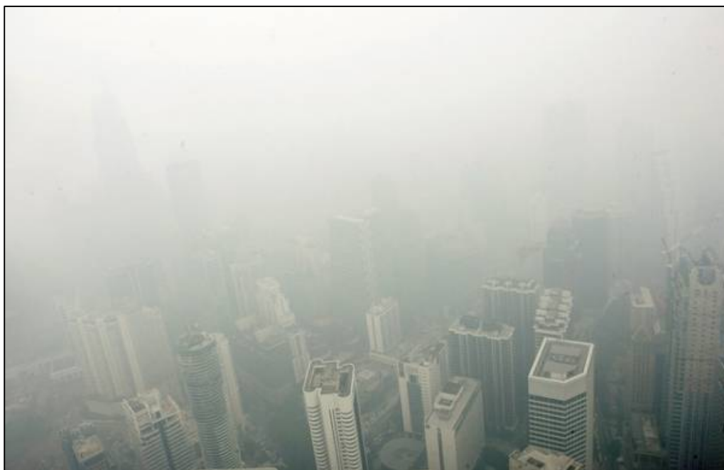
Malaysia's landmark Petronas Twin Towers and other commercial buildings are shrouded in haze in Kuala Lumpur, Malaysia, on 14 September 2015. Source: Bernama images.
