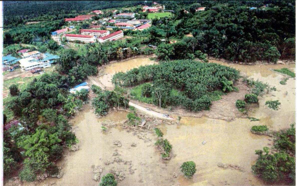
Towns in the east coast of Peninsular Malaysia and Sarawak were affected by floods last year. Flood losses can be reduced with the proper application of science and technology.
